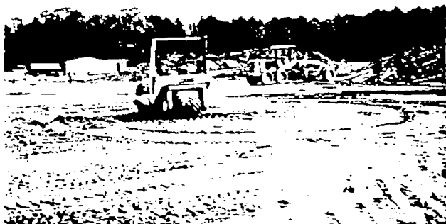
Figure 4. Fill being placed and compacted.
