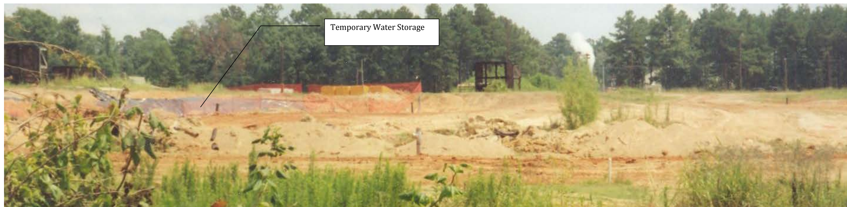
Picture 12 East of Road D Temporary Water Storage in front of BC 23S
