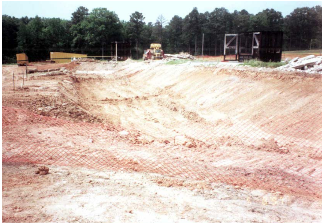
Picture 4 Along Road D looking North
