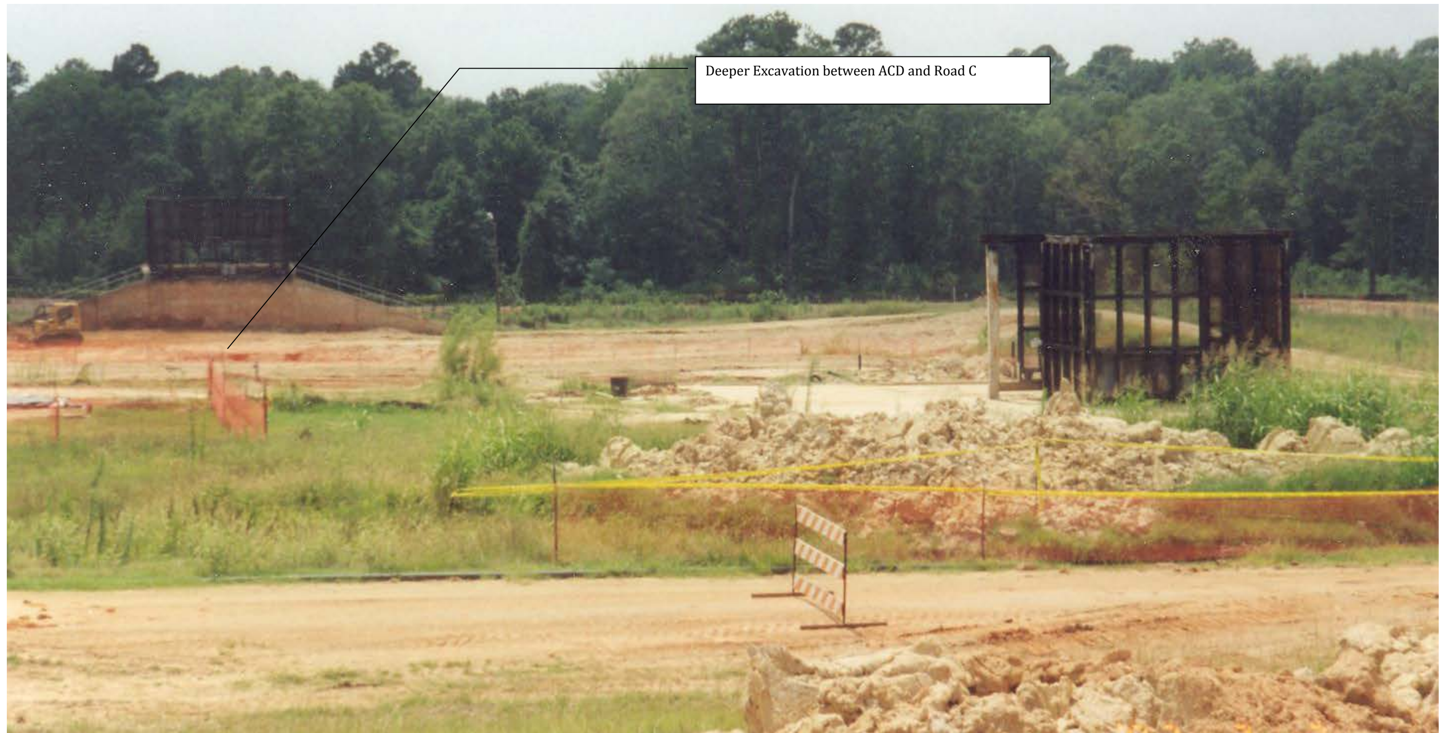
Picture 8 Excavations East of ACD
