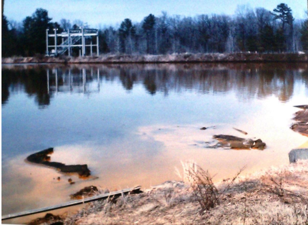
Picture 2 Unlined Evaporation pond Looking North at the Rocket Motor Washout Rack
