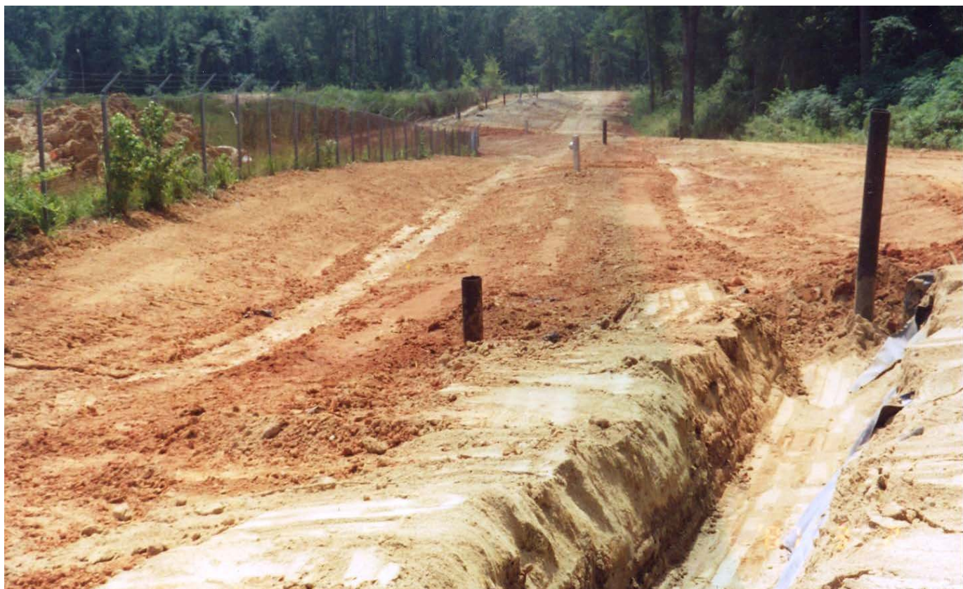
Picture 21 ICT 13 looking West Shows offset & Piezometers
