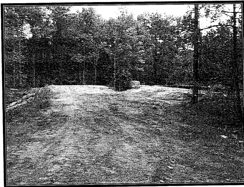
Structures after placement of fill: Building 1 on Left and Building 2 on Right
