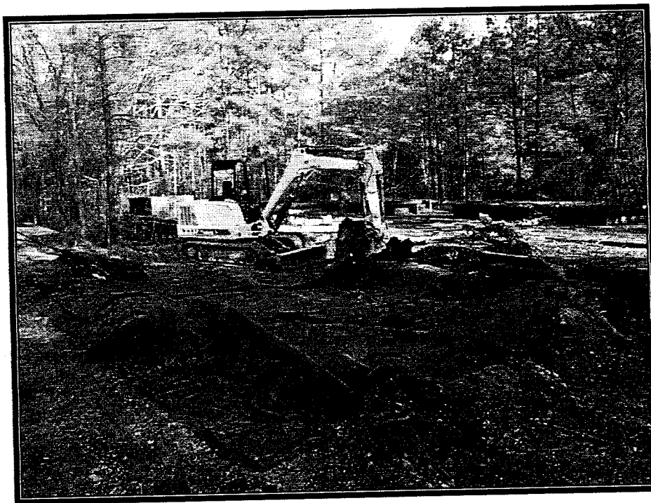
Installing Liner for Sediment Waste
