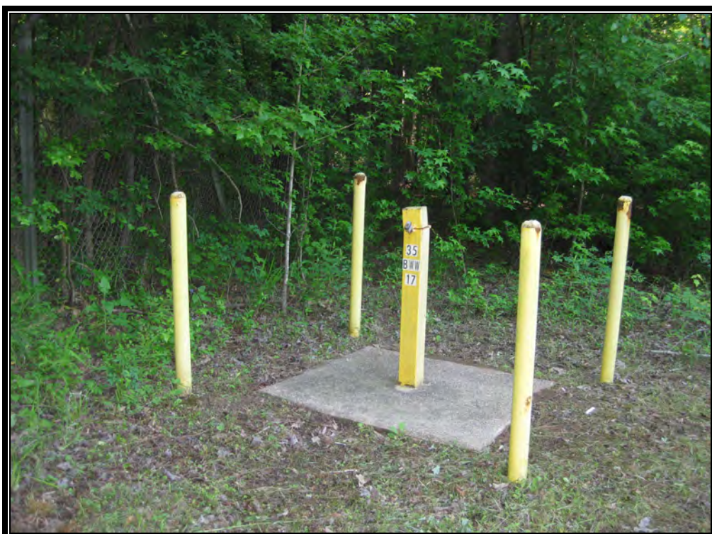
PHOTO 38: 35BWW17 DATE: May 7, 2020
