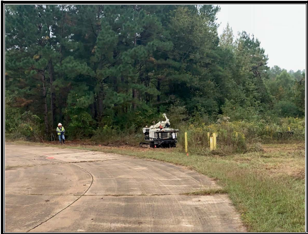
PHOTO 3: DPT Rig Setting Up to Push 04DPT17 North of Ditch and Culvert DATE: October 28, 2019
