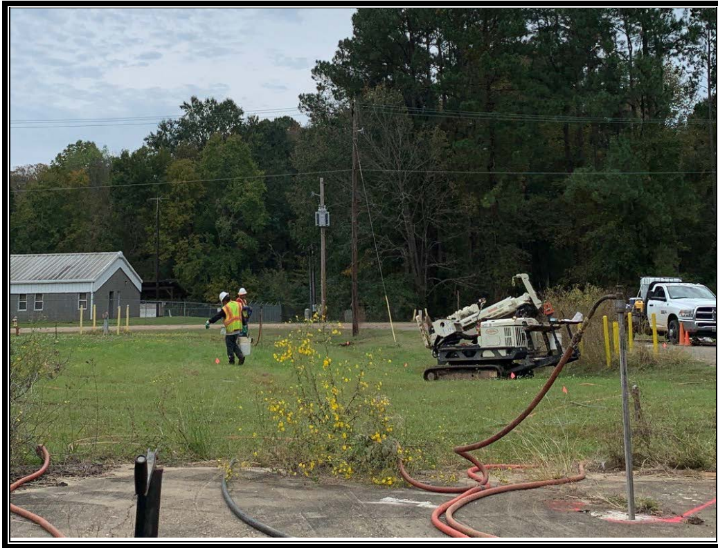
PHOTO 4: Grouting Completed DPT Locations DATE: October 29, 2019
